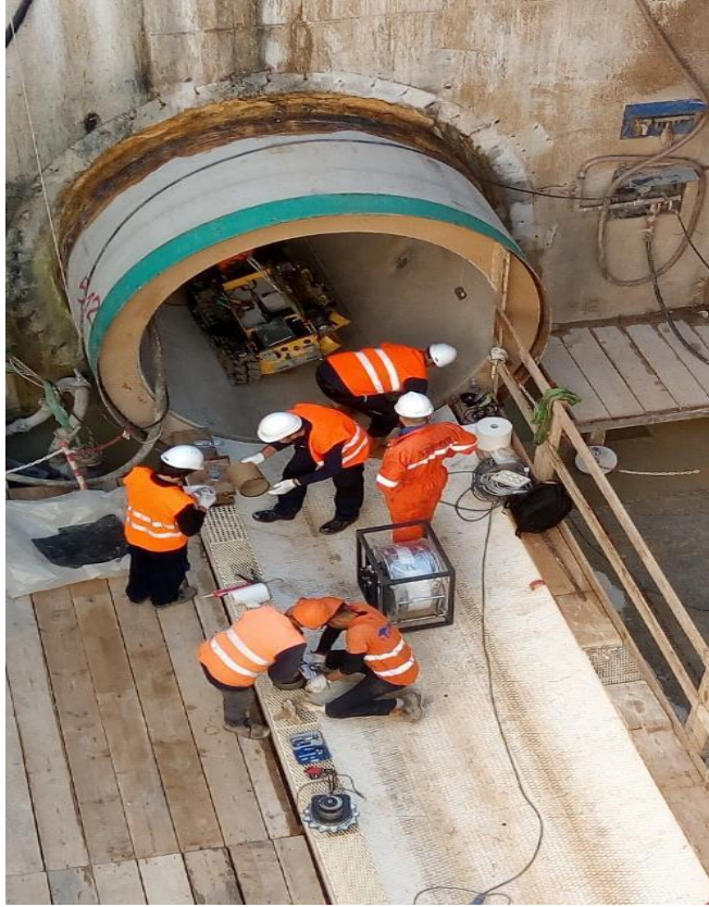
Fig 5: Electric tractor preparation for clamps and support shelves positioning
