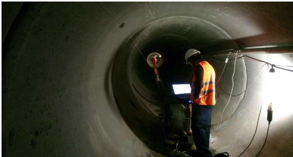
Fig 9: Monitoring system tests during installation
