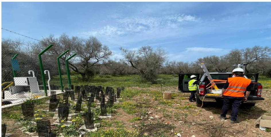
Fig 7: Microtunnel strain monitoring cabinet
