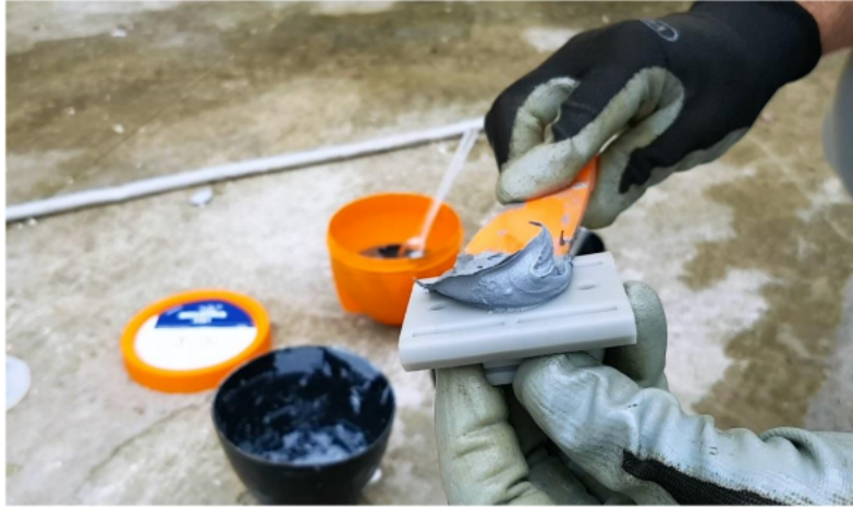
Fig 3: Application of two-component resin on the support shelf
