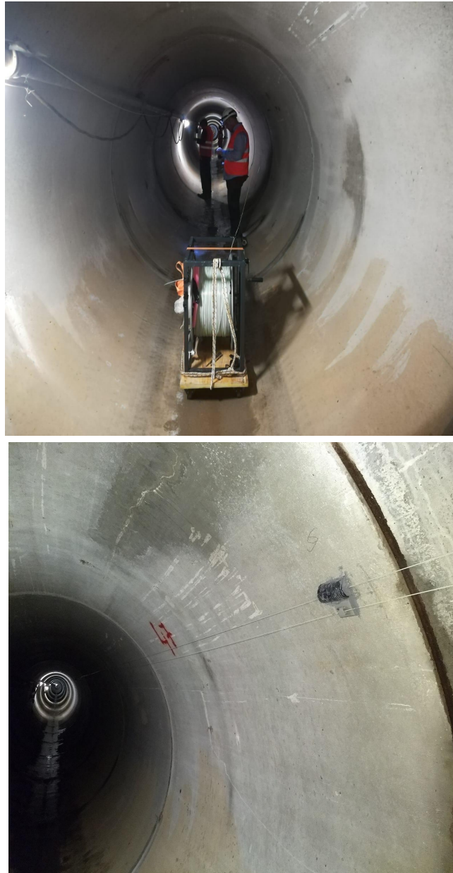
Fig 6: Sensing cables Reel for unrolling fiber optic cables (on the left) and sensing cables installation completed (on the right)
